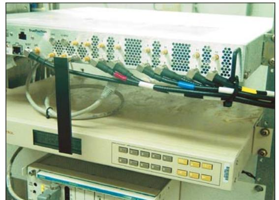
**Figure 1** · E911 location determination equipment must be reliably connected to the wireless system equipment.
